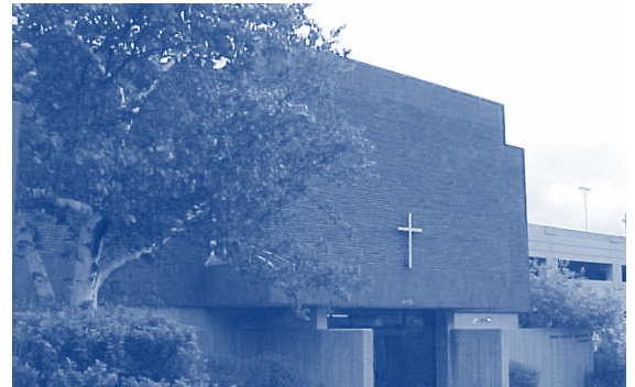
The Emma Norton Residence facility in downtown St. Paul is a 45-bed residence, offering long-term support and services for homeless women in transition, whose goals are to become independent and self-sufficient.
